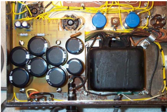
Capacitor Board Installed in Amplifier
