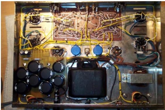
Capacitor Board Installed in Amplifier
